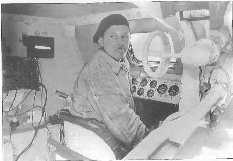
Driver's compartment in a Grant tank – see Plate G insets. The unusual hull design of the M3 Medium made this surprisingly spacious. Note the radio transceiver behind his left shoulder, and his large open front visor. This might seem enviable compared with those of other tanks; but it did let in a lot of blowing sand when on the move, and when closed down for action the driver had to peer through the usual tiny, disorienting vision slit, like that to his left. (Tank Museum 2729/E2)
